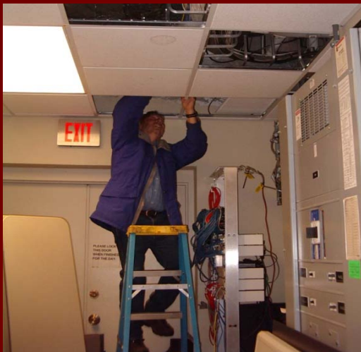
Poorly Located Heat Pumps
