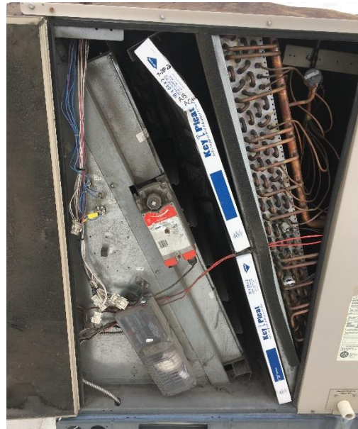
Figure 6. Picture of filter not seated correctly.
